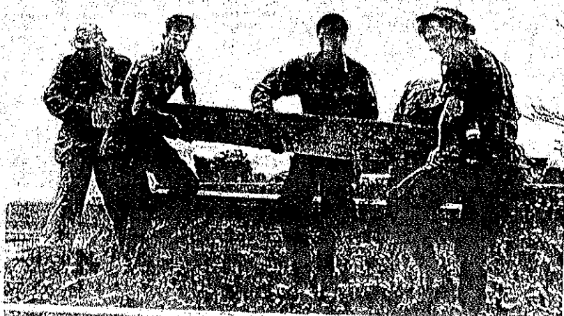
TAKING IT FROM HERE - Lt. Don Heil (far right) of Mt. Carmel, Pa., lends a hand to men of his unit, 1st Plat, A Co., 326 Engr. Bn., in building a bridge ramp. The ramp is part of the platoon's Phu Thu road project, a civic action program to open new roadways for the Vietnamese people. (U.S. Army photo)
